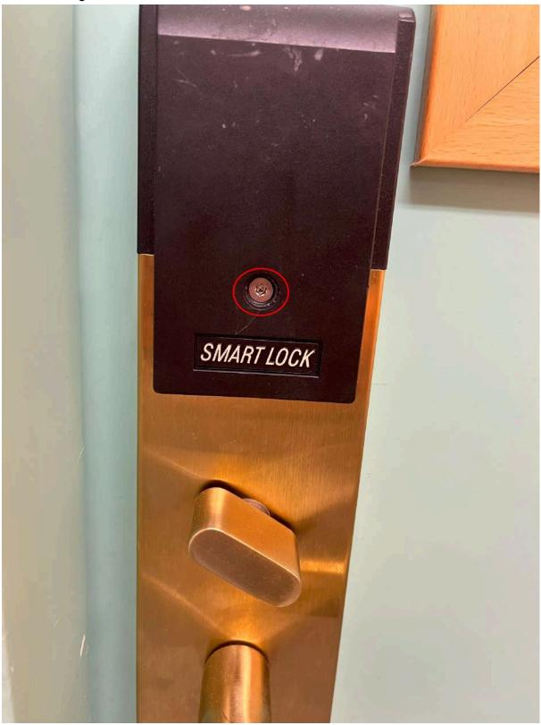
3. Disassemble the upper protective cover from the lock
